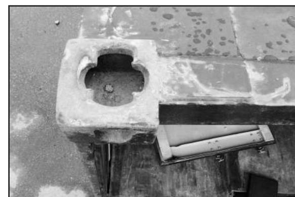
One of two failed front corner fittings on a 20' Hanjin container.
